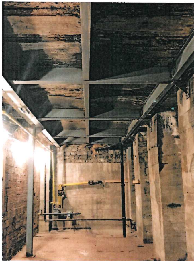
Portico Floor Deck Structural Steel Before and After
