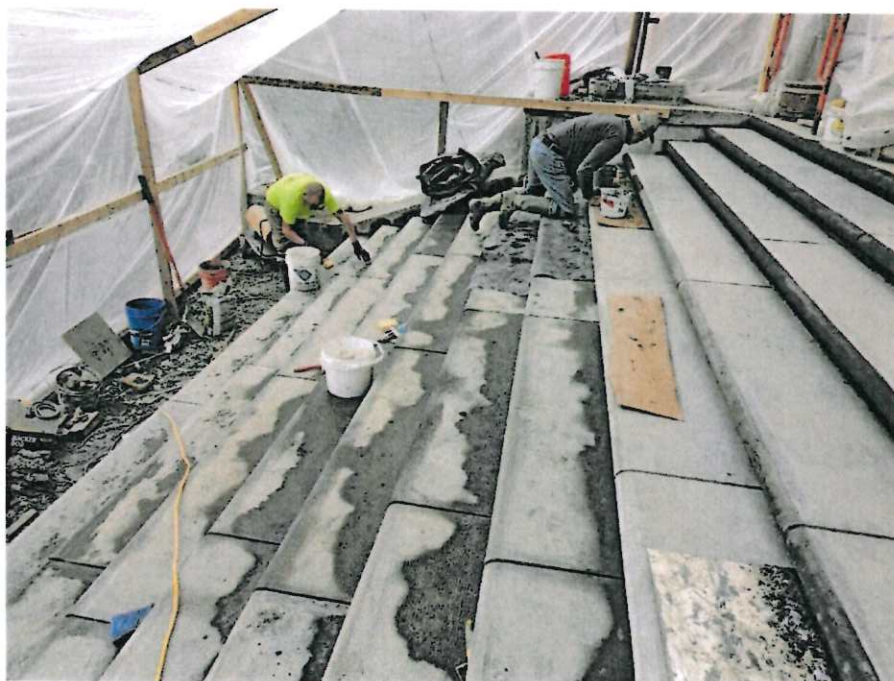
Front Steps Before and After
